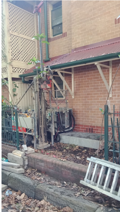
Photograph 3 – View north-east at the location of Borehole BH1.
