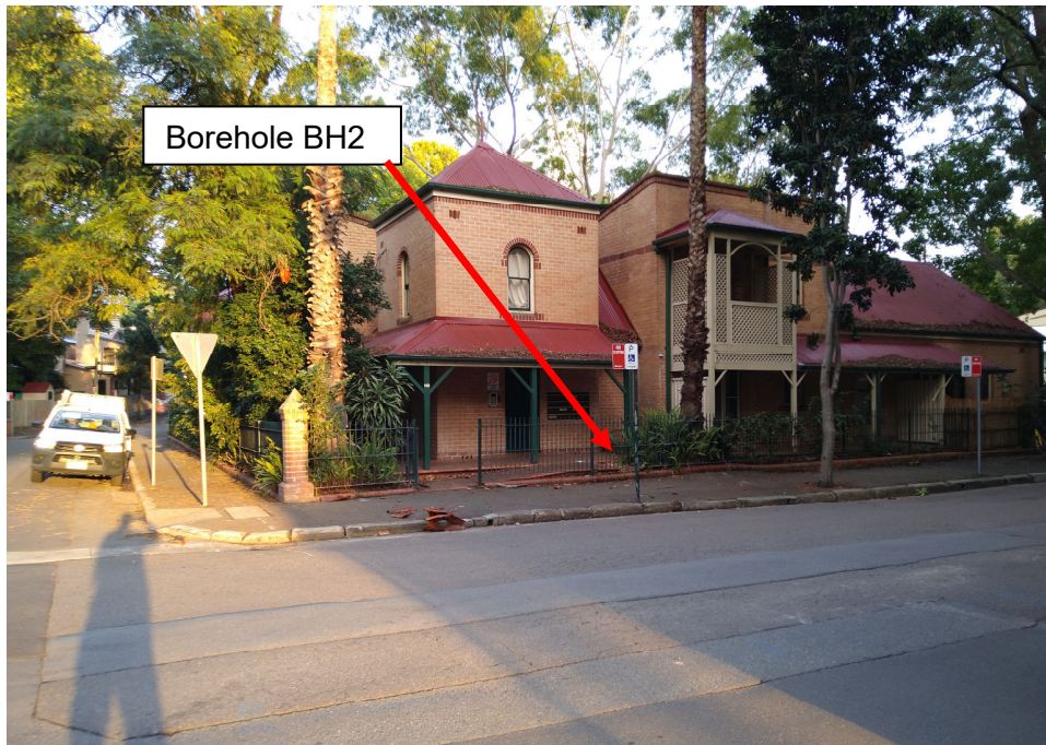
Photograph 4 – View west across Cowper Street. The approximate position of Borehole BH2 is indicated as shown.
