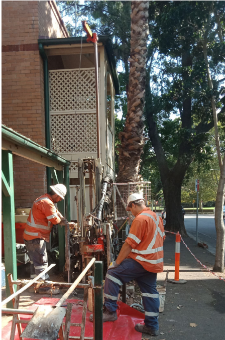
Photograph 6 – View north along Cowper Street at Borehole BH2.
