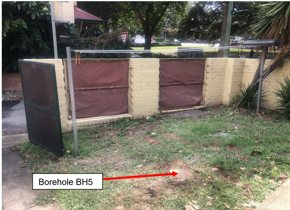
Photograph 11 – View south within the rear of the 2D Wentworth Park Road property, with Park Lane in the background. The approximate position of Borehole BH5 is indicated as shown.
